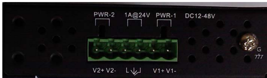
IES-2050A power connection
